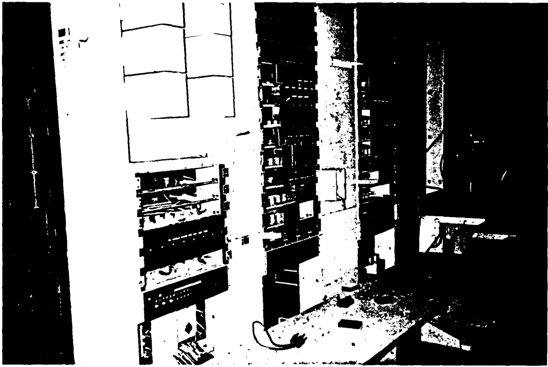
Photo 3. Electrical equipment remaining within the radio relay building.
